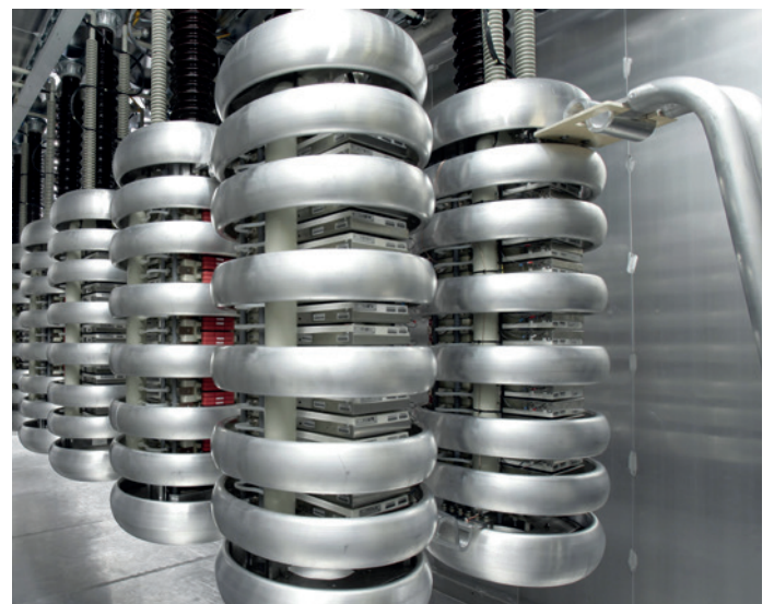
Fig. 5 Standard IGBT valve for VSC, HVDC and STATCOM
