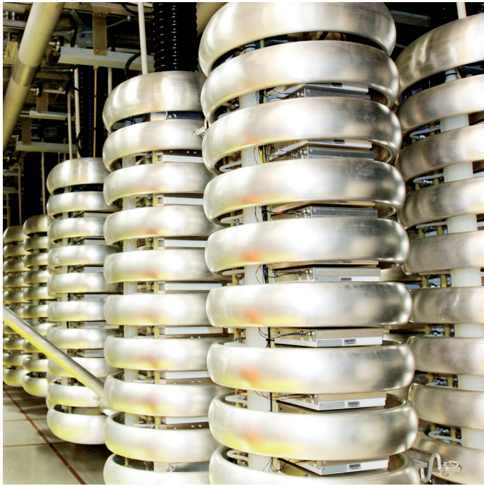
Fig. 5 Standard IGBT valve for VSC, HVDC and STATCOM
